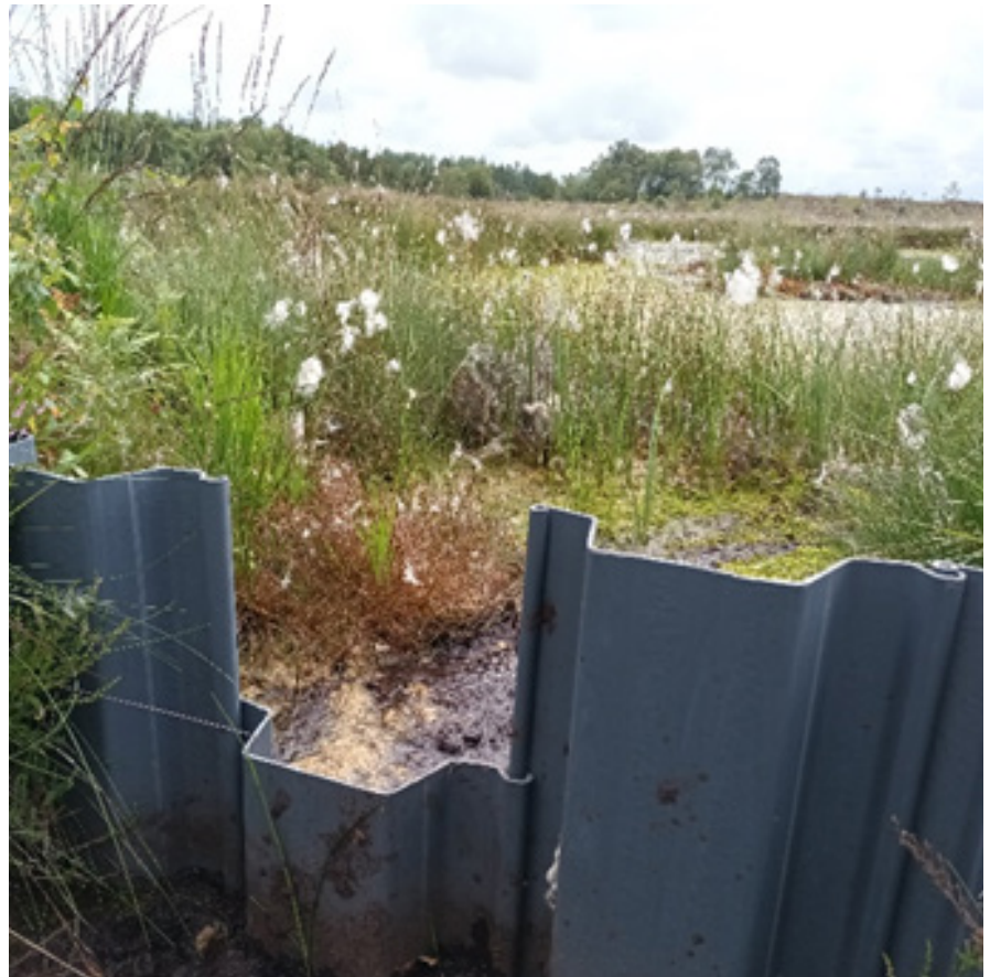
Installed Plastic Dam
