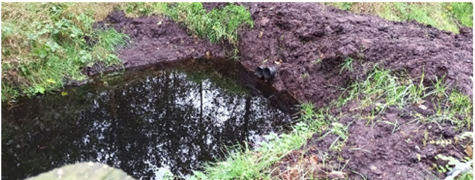
Constructed Peat Dam
