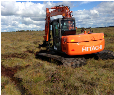
A digger doing rewetting work on Ballydangan Bog
